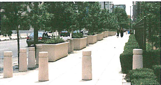
Figure 11: Concrete planters provide an attractive alternative to bollards.
