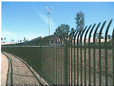
Figure 5: Fencing should be 8 feet in height.
