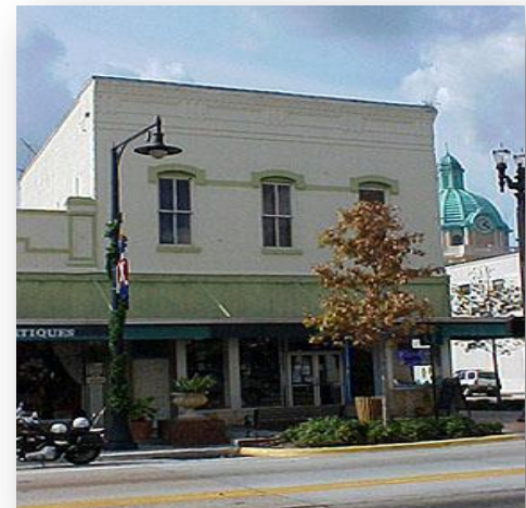
Figure 4-2 Historic Downtown Building
