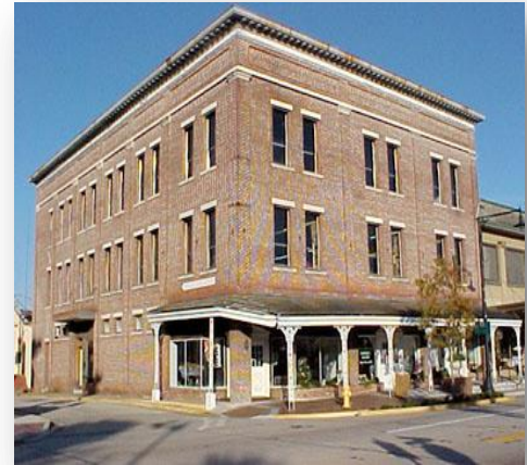
Figure 4-1 Historic Downtown Building
