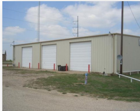
Figure 8-13 Fire Engine Bay
